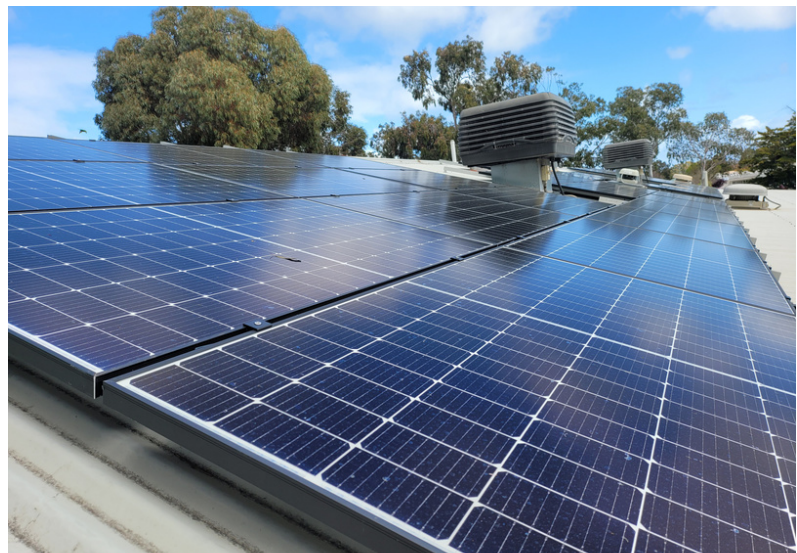
Project 43: Parkholme Community Childcare Centre
