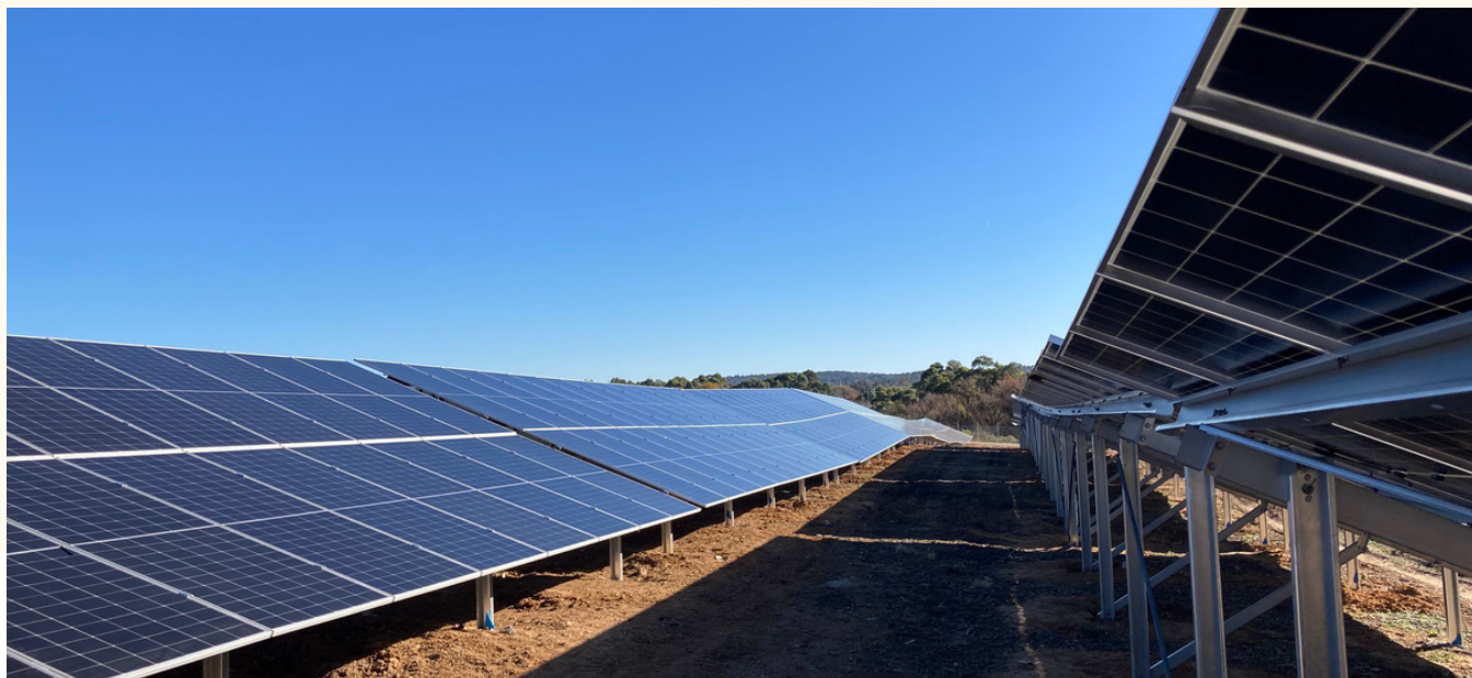
Photo Courtesy: Goulburn Community Energy Cooperative
