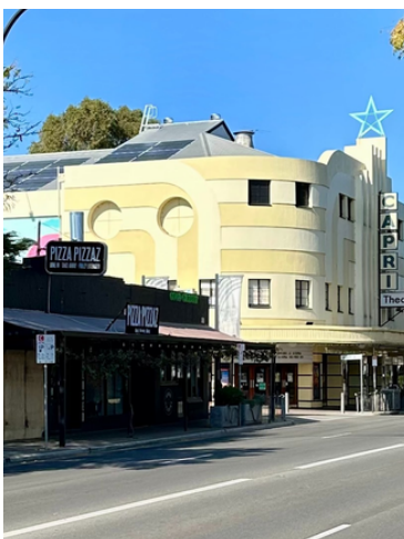
Project 52: Capri Theatre
